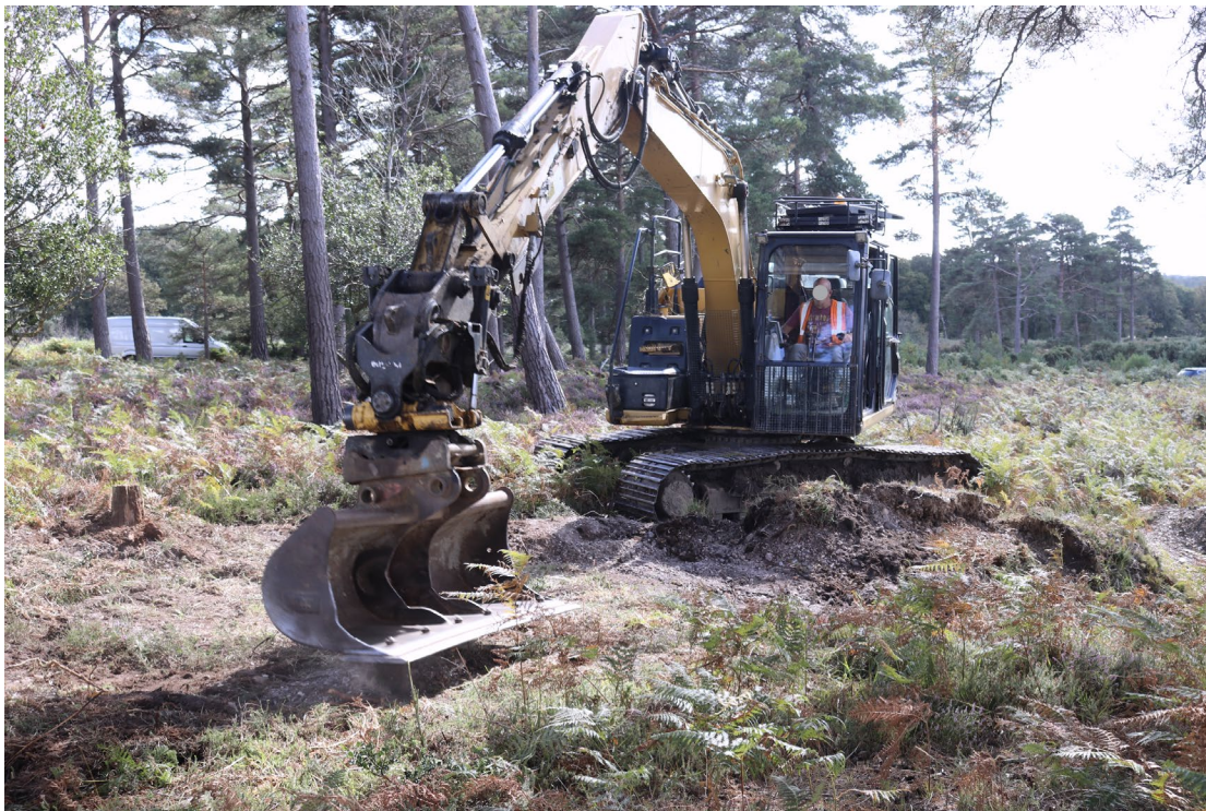
Photo 4: Working shot. Northern end of eastern boundary earthwork.
