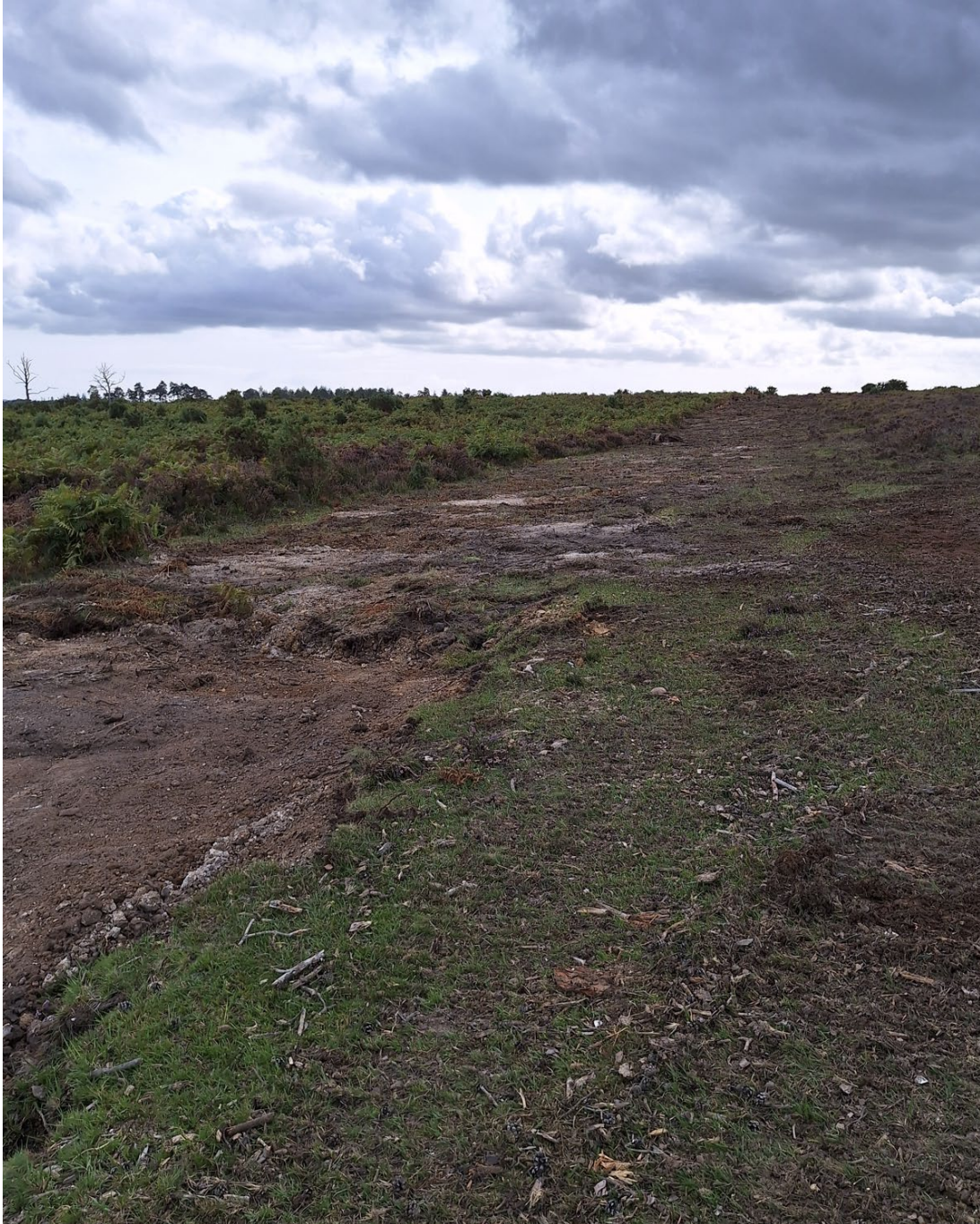
Photo 12: Southern end of eastern boundary earthwork, post levelling, looking S.
