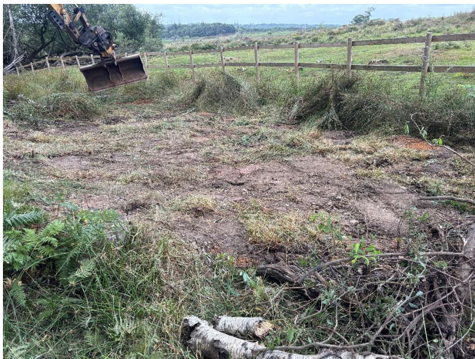
Photo 7: Working photograph of the final surface (looking W).
