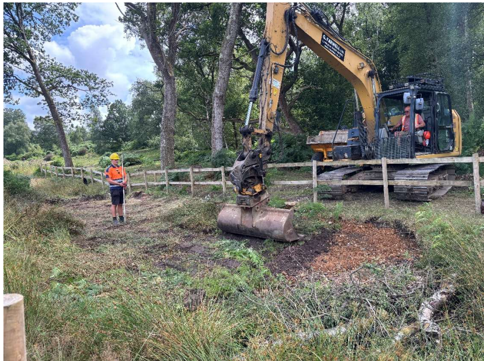
Photo 5: Working photograph of turf reinstatement (looking SE).
