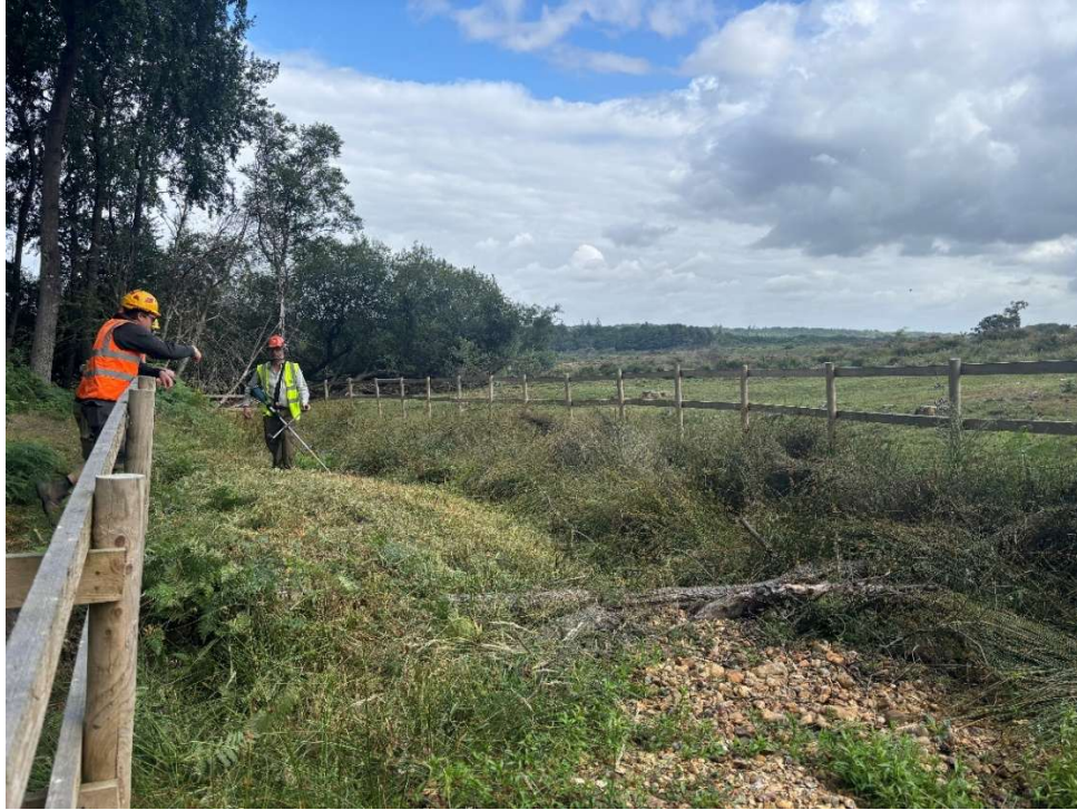
Photo 2: Ground preparation prior to machine excavation (looking SW).
