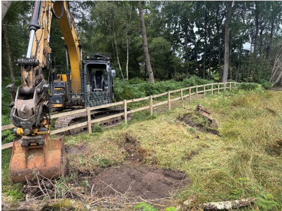
Photo 3: Machine excavation of the enclosure bank (looking S).
