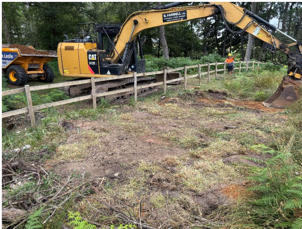
Photo 6: Working photograph of the final surface (looking S).
