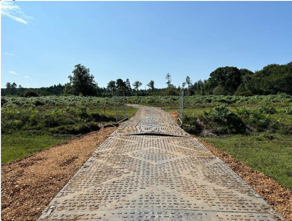
Photo 1: Established protective surface crossing Bishop's Dyke and temporary roadway, 2024.
